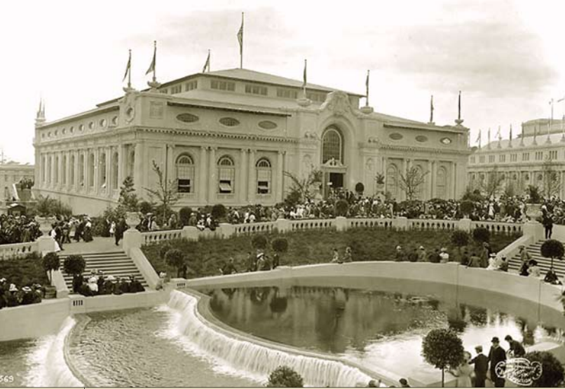
ABOVE: The Alaska Building, one of the exposition's centerpieces, showcased the wealth and resources of the territory to the north. University of Washington Libraries Special Collections
